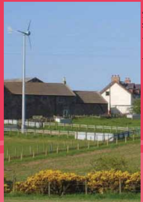
Image courtesy of Aegis Energy
